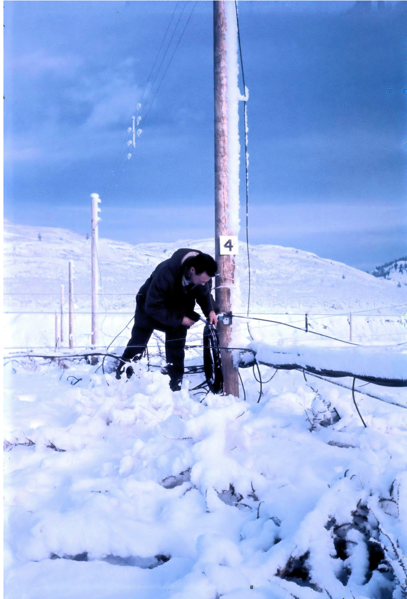
Mike Robinson working at the 10-MHz array's most common failure point – soldered joints at the individual dipole baluns, which needed constant monitoring
