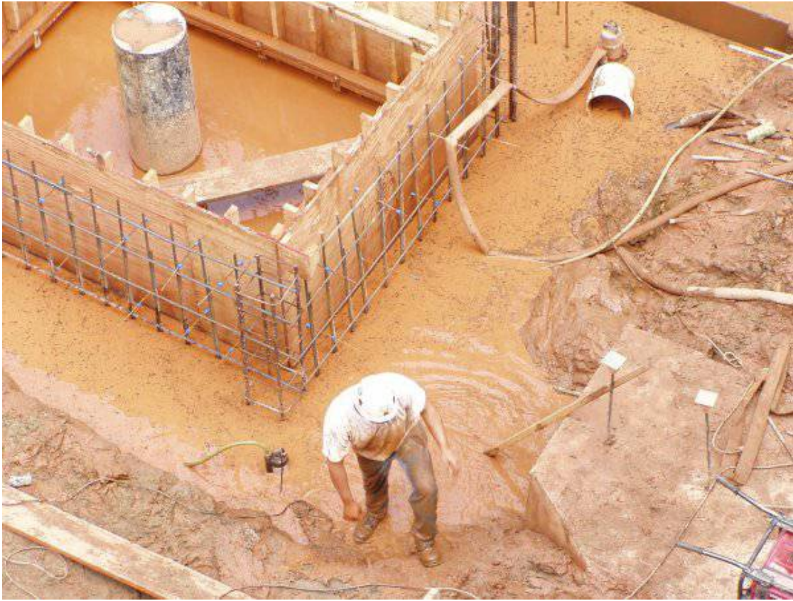
The "Summer of Mud": construction around the elevator jack in August 2003
