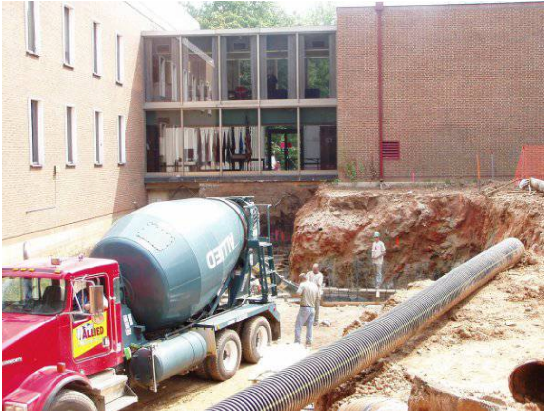
First concrete was poured for footings of the Addition on July 15, 2003
