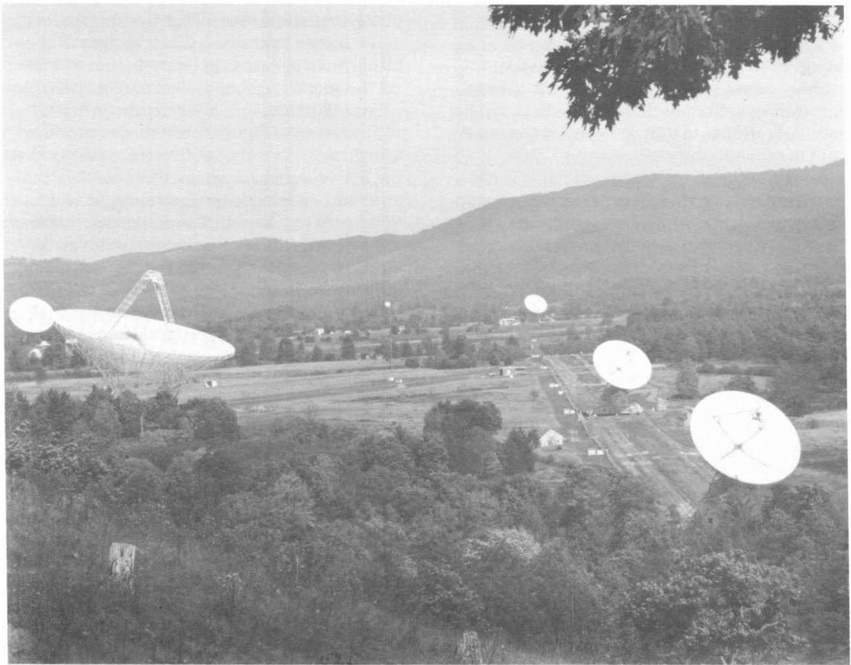
Figure 3. General view of the Deer Creek Valley, containing the National Radio Astronomy Observatory's site at Green Bank, Virginia. The 300-foot antenna shown in Figure 2 is in the foreground to the left. The smaller (85-foot) antennas stationed in a line to the right of this view are used together as a three-element interferometer. As described in the text, these three antennas are moved both by the Earth (which rotates the whole scene around once per day) and also by relocating them along the runway that joins them, to build up the information that would be collected instantaneously by radio telescope about twice the size of the valley.
