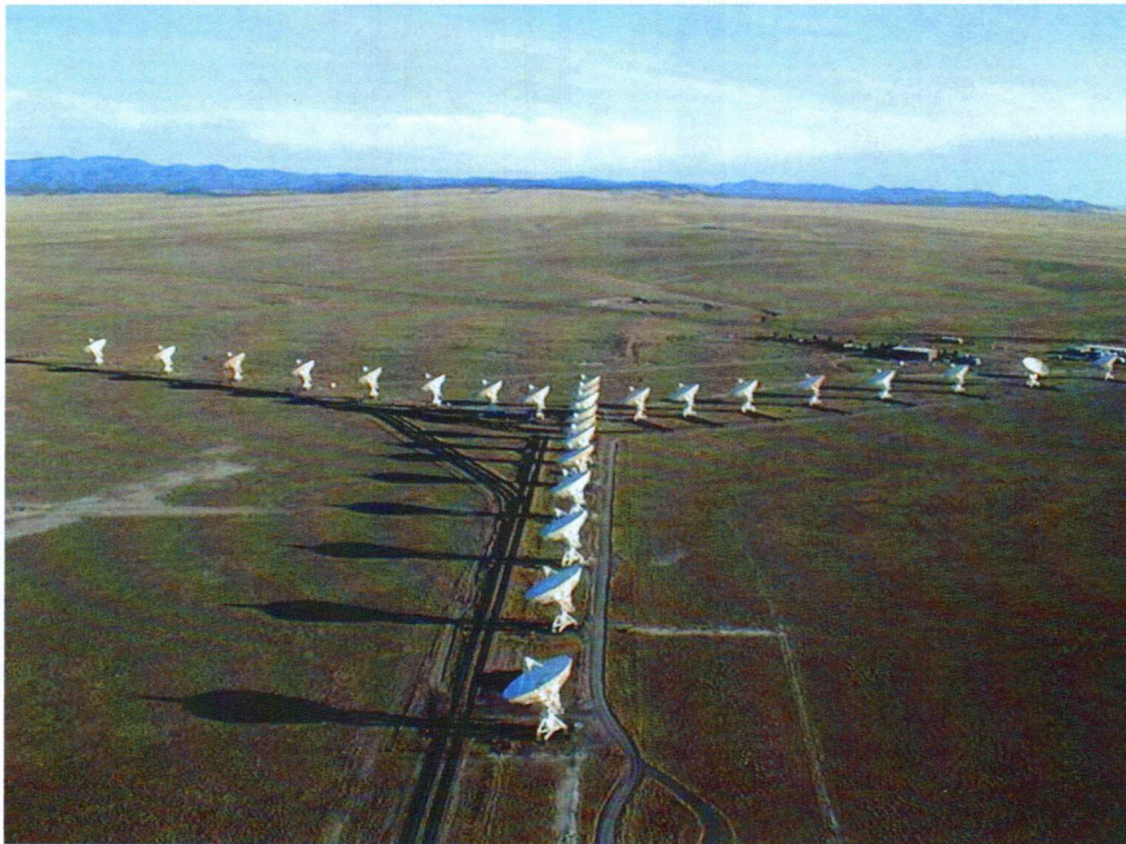
FIGURE 12.3 The NRAO's VLA on the plains of San Agustin near Socorro, New Mexico. The VLA uses 27 25 m (82 ft) antennas to make images of the radio sky at centimeter wavelengths by Earth-rotation aperture synthesis. (From © NRAO/Associated Universities, Inc.)
