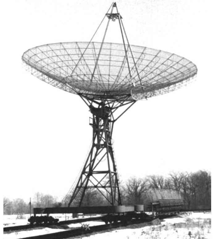
Figure 10 — The QRO 18-m dish on E-W rails in 1969. Plans for a second dish to form an interferometer were never implemented. In the background to the East sit the twin arrays for 35cm wavelength built by the Electrical Engineering Department.
