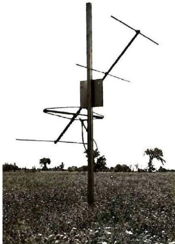
Figure 1 – Half of Queen's University's first radio telescope at Westbrook in 1958—one of two Yagi antennas comprising Arnold Matthews' east-west interferometer for recording scintillations of Cas A at 6m wavelength. The three metal rods (one "reflector" dipole and two "director" dipoles) are 3m long. The diamond shape (a dipole "folded" to raise its impedance) is connected by coaxial cable to the receiver in a central hut. The loop of cable hanging down (a "balun") prevents currents from flowing on the outside of the cable and disturbing the shape of the Yagi's reception beam (its "power pattern").
