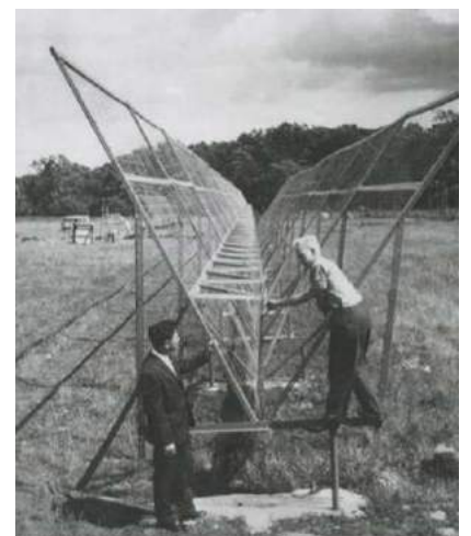
Figure 6 — The long E-W fixed arm of the 2m “moving-tee” synthesis telescope, under construction in 1962. The beginnings of the moving element are visible to the left. Professor George Harrower stands, while Philipp Kronberg climbs on the 60-degree corner reflector. Kronberg is holding one of the 96 end-to-end folded dipoles that together form a “line feed” for the corner reflector. The sides of the reflector are wire mesh, which acts as a mirror for radio waves. With mirrors 60° to each other, 5 images appear. The real line feed plus its five images act together as an array of long antennas, increasing the sensitivity of the telescope to incoming waves.
