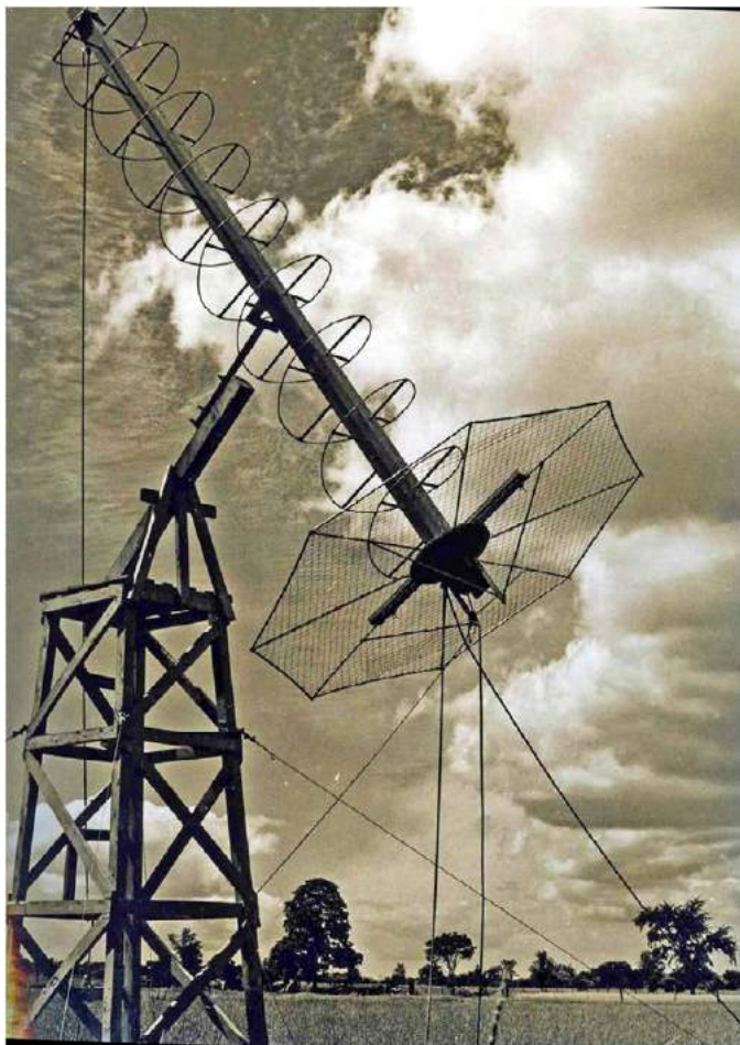
Figure 2 — David E. Hogg's M.Sc. project—studying transient bursts of radio noise from the Sun by scanning repetitively in wavelength from 3.4m to 2.3m at 5-second intervals. The antenna is an equatorially mounted 9-turn helix of length 6m, with a reflector of diameter 3m. The receiver output is recorded directly from an oscilloscope screen by a camera.
